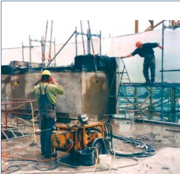
Diamond sawing in Wuppertal
