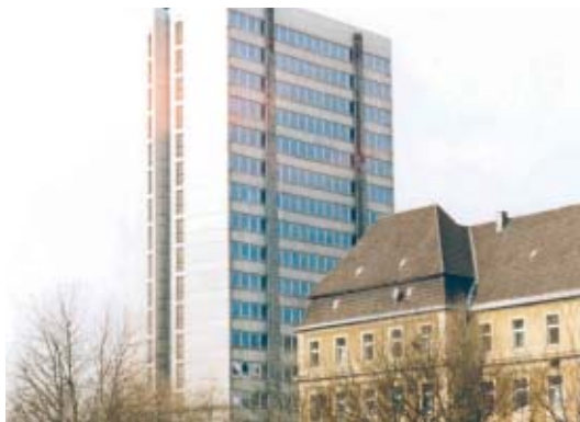
Wuppertal courthouse prior to demolition
