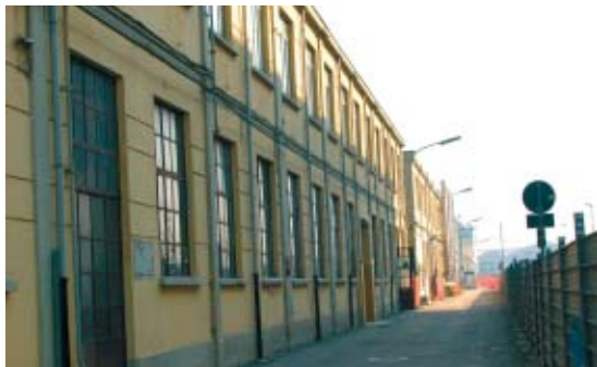
Pirelli building prior to demolition
