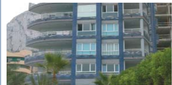
Aluminium identified in windows and balcony fences in Alicante
