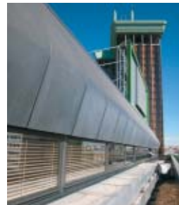
Aluminium cladding, windows and ducts
