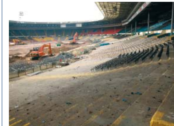
The stands after removal of all the seats
