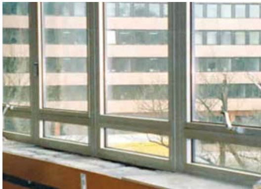
Aluminium window frames in the Wuppertal courthouse
