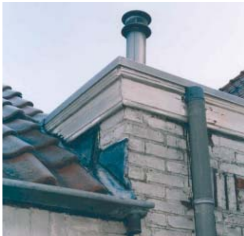
Aluminium identified in roof strips and chimneys
