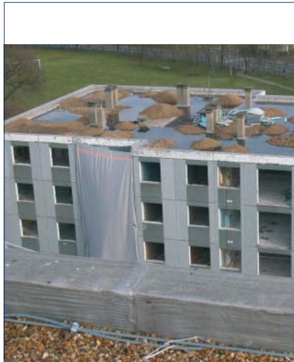
Apartment building in Le Mans during deconstruction and demolition
