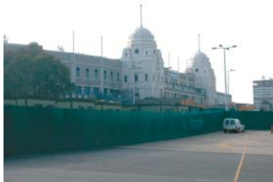
The famed Wembley twin towers prior to demolition
