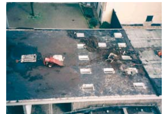
Removal of hazardous waste from the roof of the courthouse
