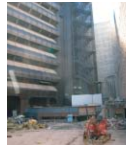
Demolition in progress
