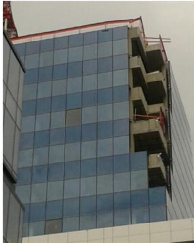
**Figure 1: Installation of a curtain wall**
